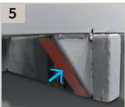
Main frame triangular reinforcement brace added
